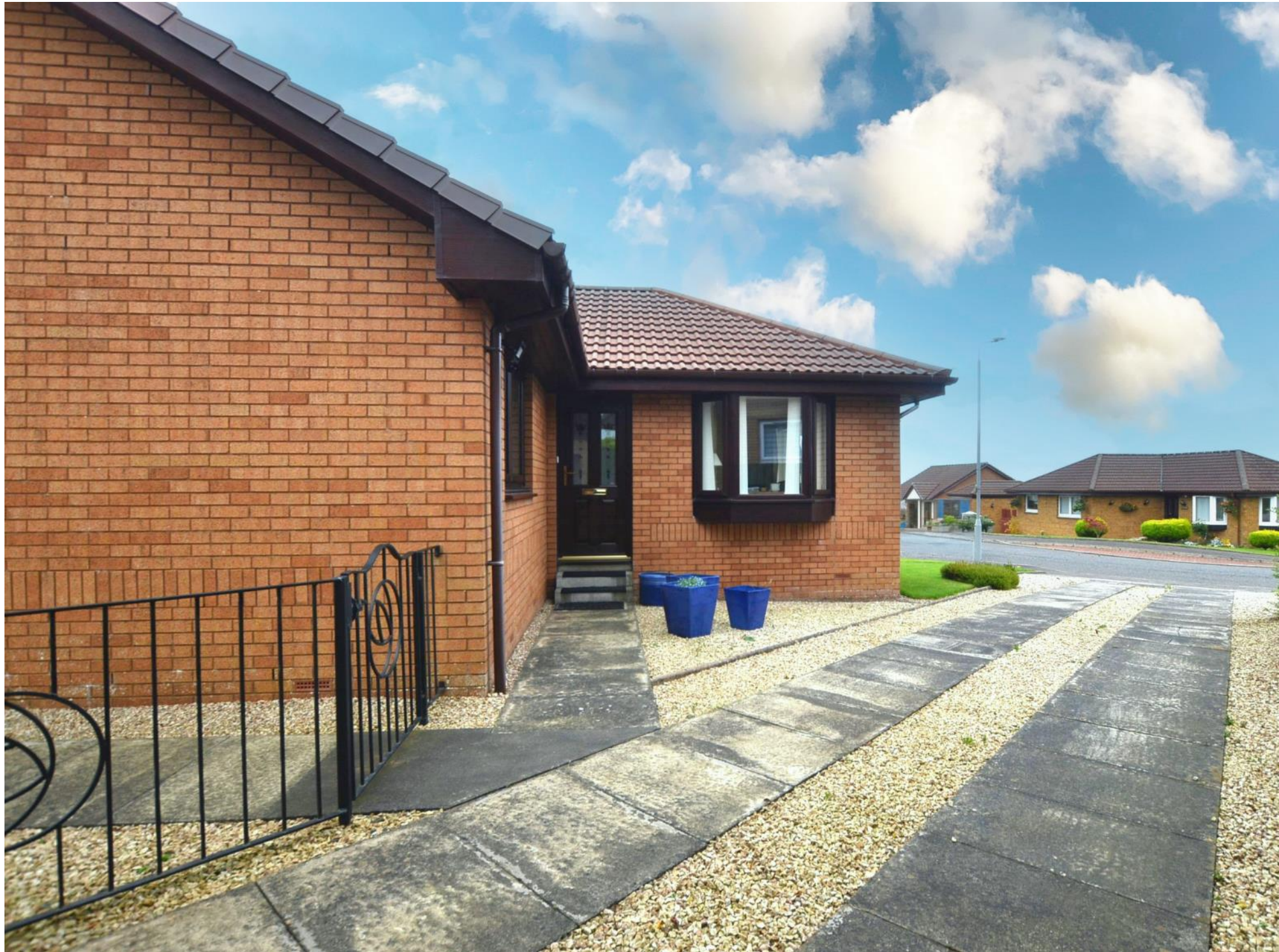
Below: Front of Property
